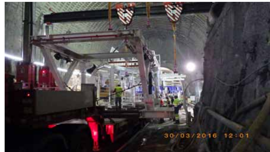
Montage tunnelier Federica
