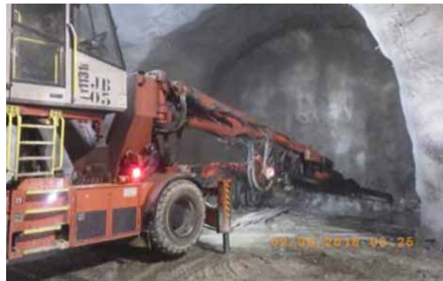
Saint-Martin-la-Porte Niche PM 1450- Foration du front
