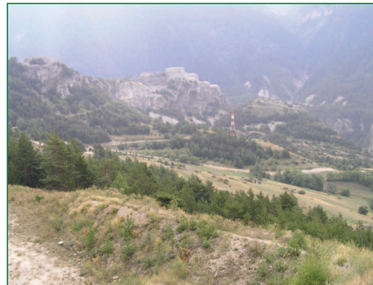
Forts dominants le site (Scetauroute 10/09/04 et 21/07/04).
